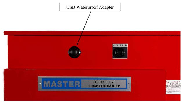
To read the data from the USB, simply plug in the USB into any computer and open the CSV file with any spreadsheet program.
